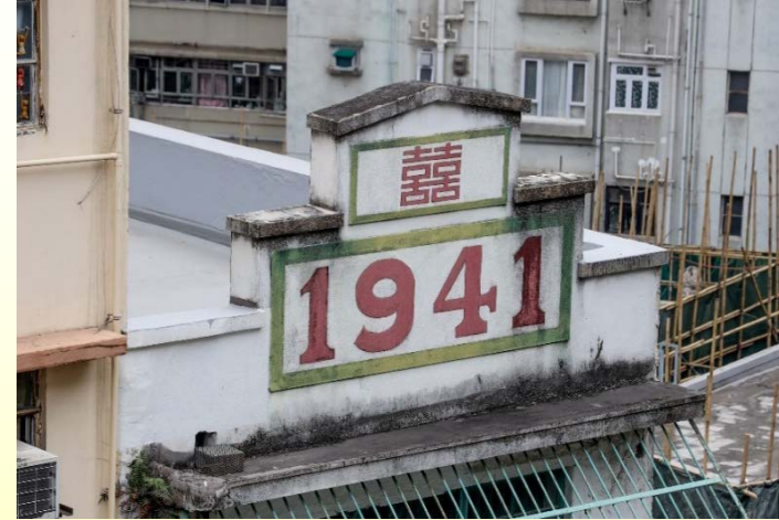
屋頂矮牆 Parapet at roof
